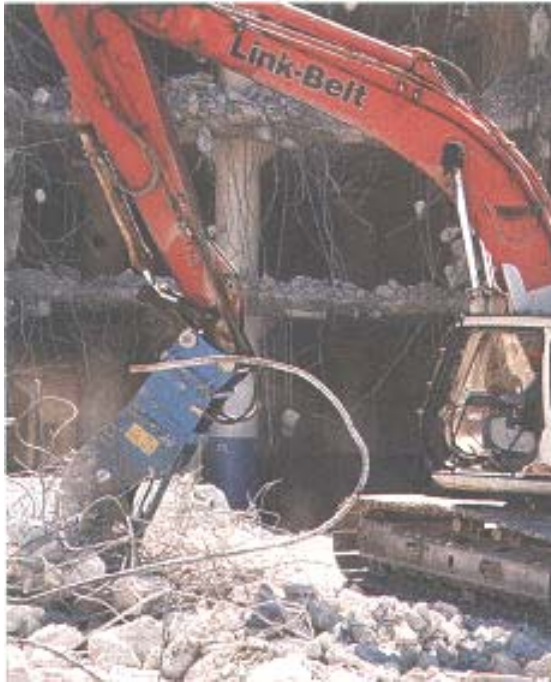
↑Conventional and implosion demolition
