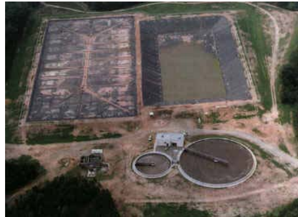
Wastewater Plant at Poultry Processing Plant in N.C.↑
