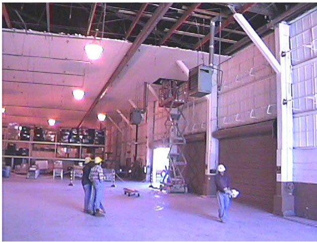
↑Removal of Hanger Ceiling at Randolph A.F.B., TX.
