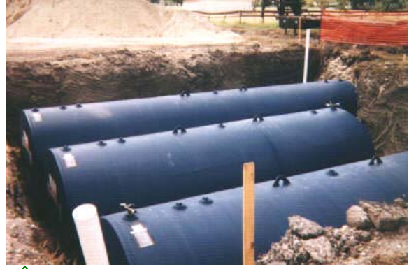
↑New USTs Installed at Exxon Station in Vanderbilt, TX.
