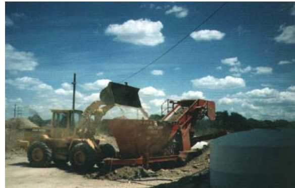
On-Site Bioremediation at Manufacturing Facility ↑
