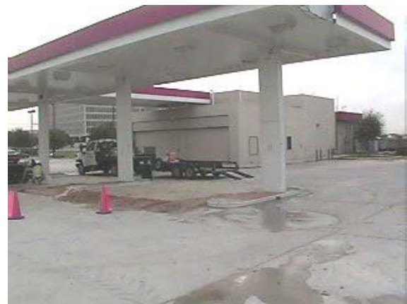
Tank System Closure at Exxon Station, San Antonio, TX ↑.
