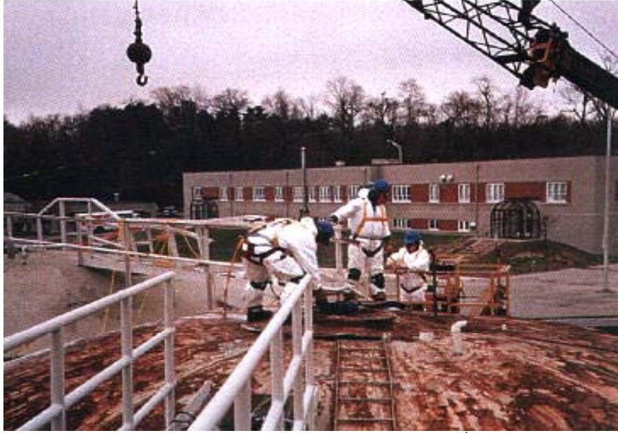
Plant Dismantling and Recycling at Manufacturing Plant ↑
