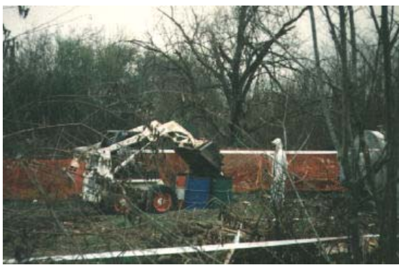
↑Hazardous waste removal and disposal
