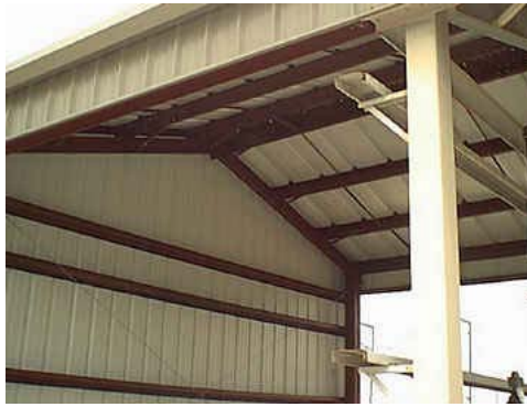
↑Canopy Construction at Judson I.S.D. Transportation in Converse, TX.
